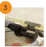
Mounting bracket available for in-roof applications
