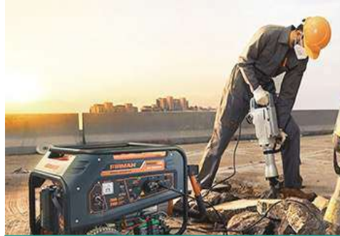
Power Generation Equipment
